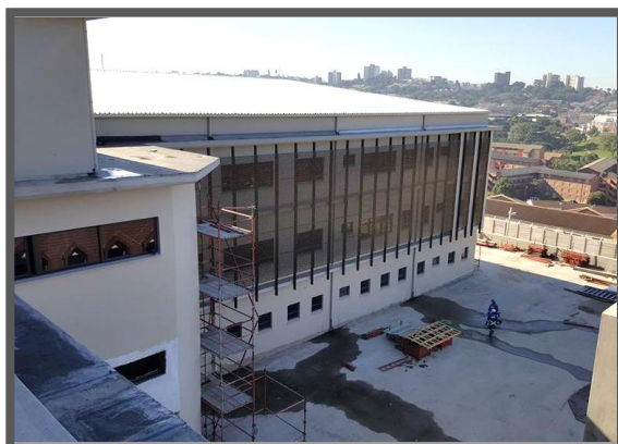
The installation of the screens has started.
