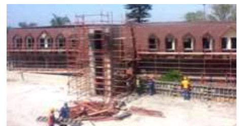
Mansard Building currently being upgraded including a new lift
